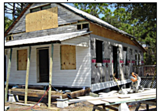
#5 Rafters and new siding
