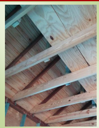
Interior Ceilings are also awaiting completion
