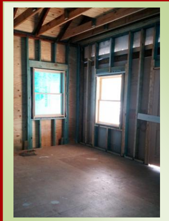
Interior Walls still need to be completed.
